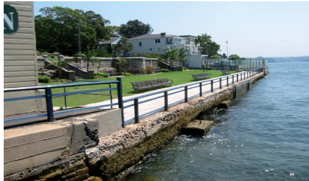
Above: Existing seawall on Thornton Park frontage has been recently repaired. The type of repair is unsympathetic to the heritage significance of the seawall and should not be replicated at the 2 - 8 Weston Street site.
